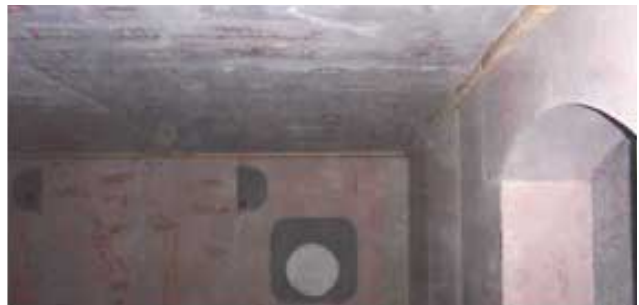
Typical furnace installation showing lower wall, upper wall and roof
